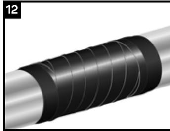
Allow SCG to reach a Shore D Hardness of 60 prior to pulling. SCG is fully cured at a Shore D Hardness of 80 at 23°C (72°F).
