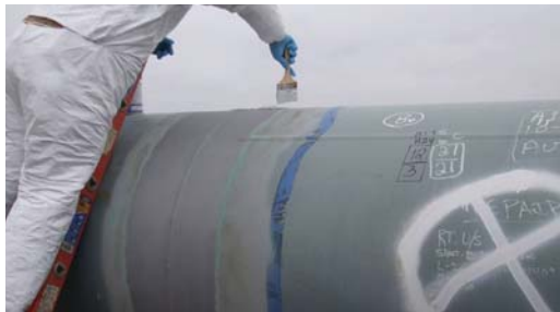
Applying Protal 7125 by brush.
