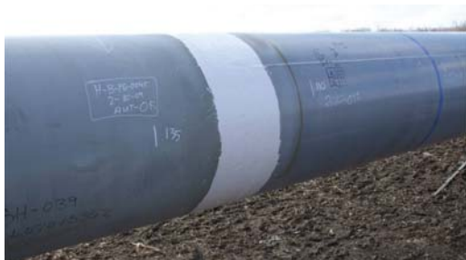
Coated girth weld with Protal 7125.
