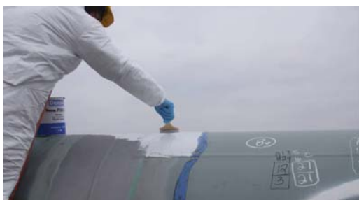
Applying Protal 7125 by brush.
