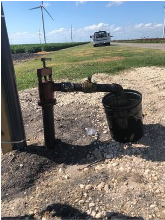
Figure 3. Casing Fill Hook-Up Equipment With 5-Gallon Bucket.
