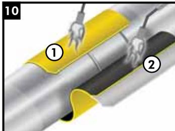
Wrap the sleeve loosely around the pipe, ensuring the appropriate overlap. Gently heat the backing of the underlap and the adhesive side of the overlap.
